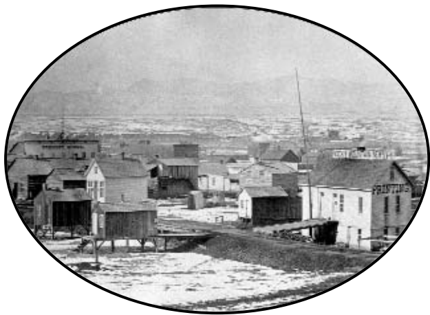
Byers' Rocky Mountain News Building
