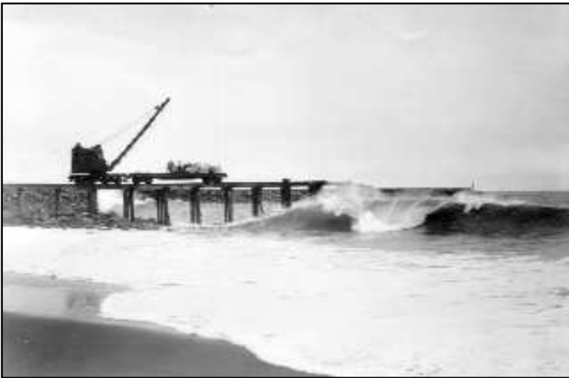
Building of Rock Groin West of Jetty
